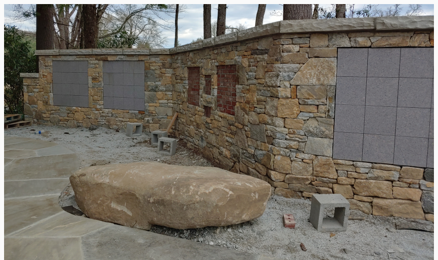
MEMORIAL GARDEN WALL WITH NICHEs
